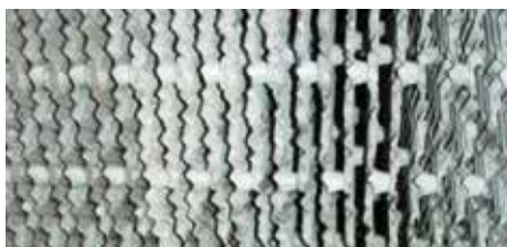
Before Vulcan was installed: the inside of the cooling tower.
