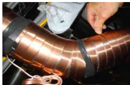
Vulcan Impulse Cables double wrapped on water pipe
