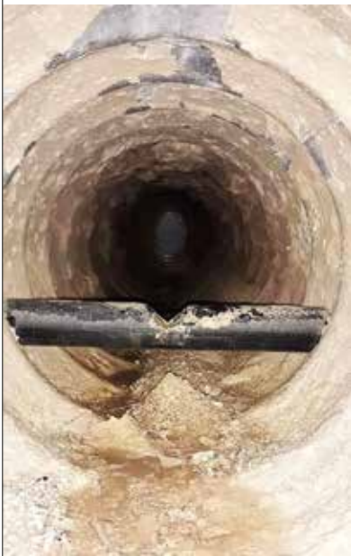
After Vulcan S25 had been installed for 6 months , the boiler was opened: scale had been softer and left out.
