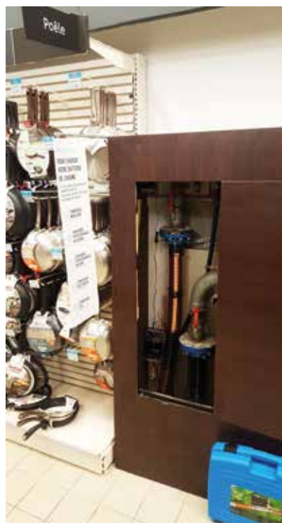
Vulcan S25 was installed in the water main to treat the whole building.
