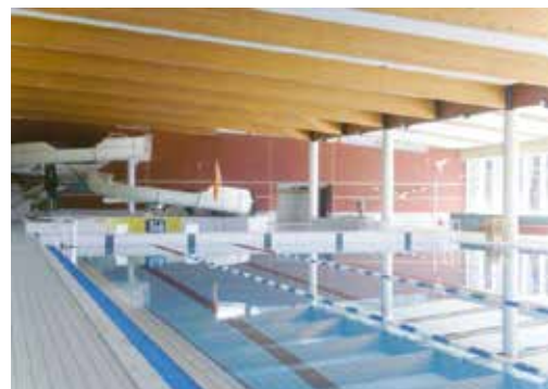
Swimming pool and water slide inside the Centre Nautique
