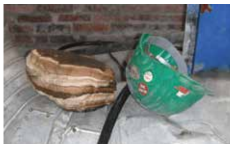
Deposit removed from pipe after Vulcan installation
