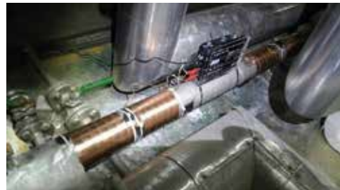
Vulcan S25 installed at Toray Industries
