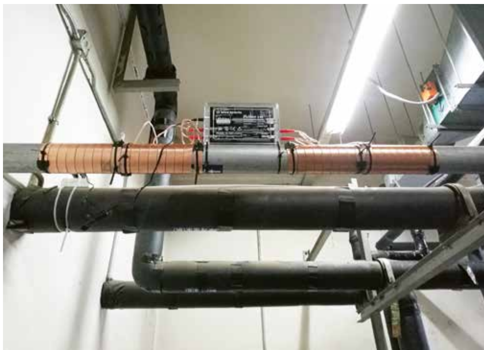
Vulcan S25 installed on the main water pipe of the cooling tower.
