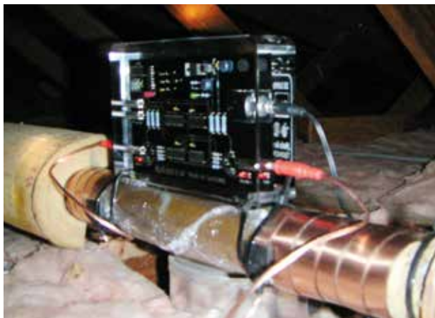
Vulcan S10 installed on water main for Bodega housing dormitories
