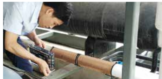
Installing Vulcan S100
