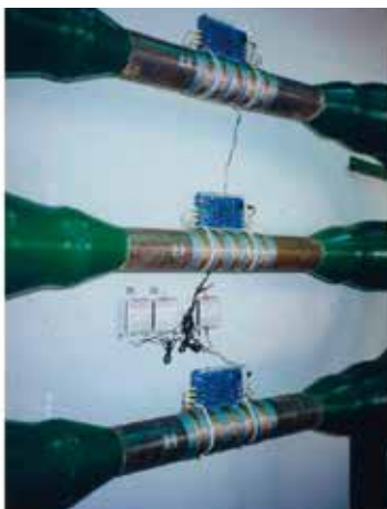
After Vulcan installation
