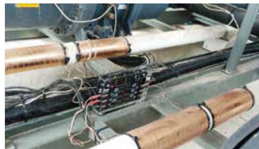
Vulcan S100 was installed on the main air-conditioning system
