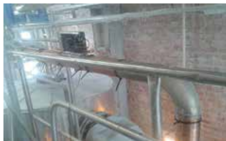
Installation of Vulcan S100 on lime kiln
