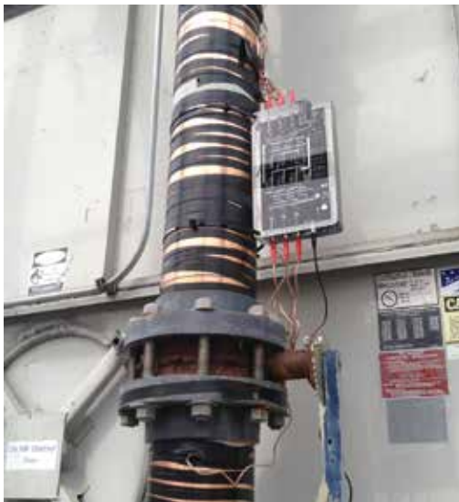
Vulcan S100 installed on cooling towers
