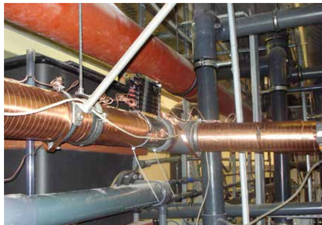
Vulcan S250 treating main water pipes for the Meridan Pool and Spa area
