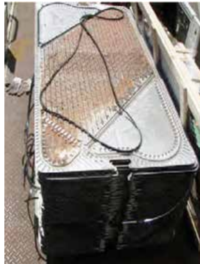
After Vulcan was installed for 9 months: the plate heat exchanger was taken apart for cleaning.
